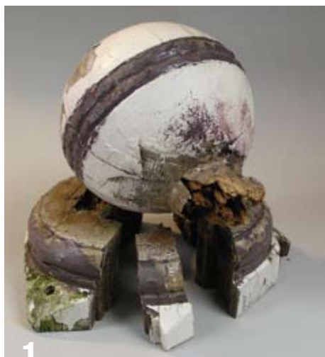
1 Original newel post cap, rotted.
